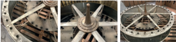
The fittings were in poor condition after years in storage.
