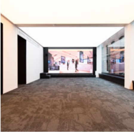
Stretched ceiling incorporating digital graphics, to create art and various light scenes.
